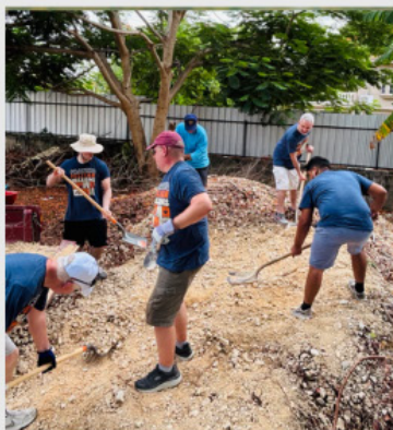
Sidewalk Building in San Ignacio, Belize
