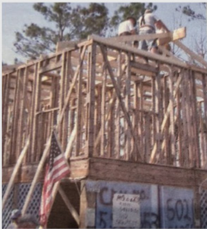
Rebuilding after Hurricane Katrina - Our Lady of the Gulf Parish, Mississippi
